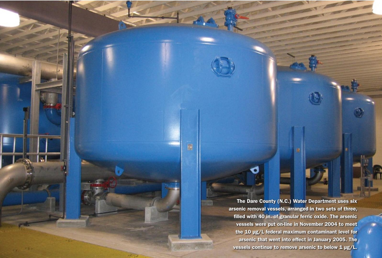
The Dare County (N.C.) Water Department uses six arsenic removal vessels, arranged in two sets of three, filled with 40 in. of granular ferric oxide. The arsenic vessels were put on-line in November 2004 to meet the 10 µg/L federal maximum contaminant level for arsenic that went into effect in January 2005. The vessels continue to remove arsenic to below 1 µg/L.
